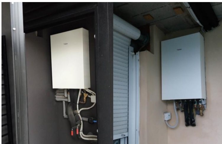
Image 36: transfer modules Antzieta 12 and 22
