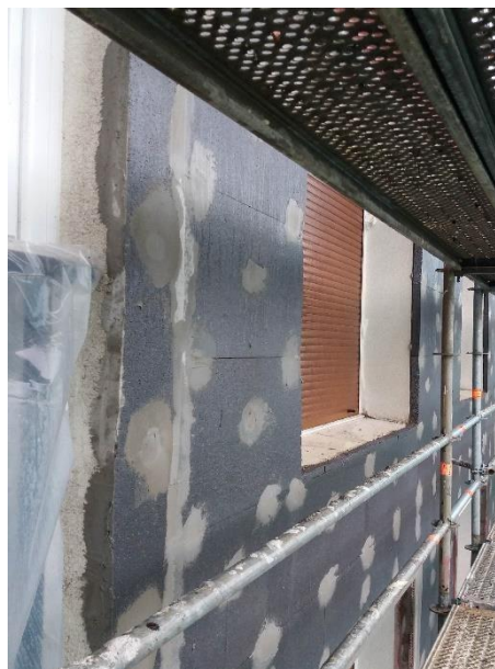
Image 10: thermal insulation SATE system
