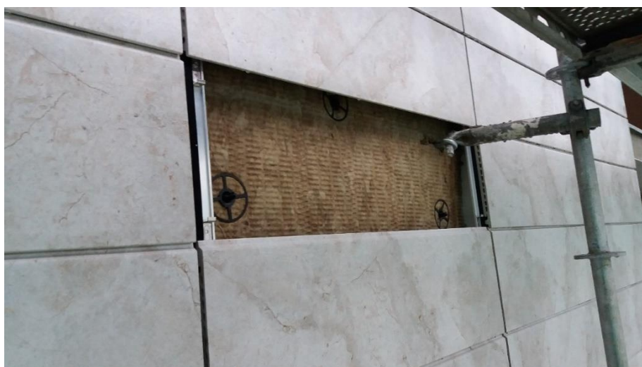
Image 16: Antzieta 31 Ventilated façade detail
