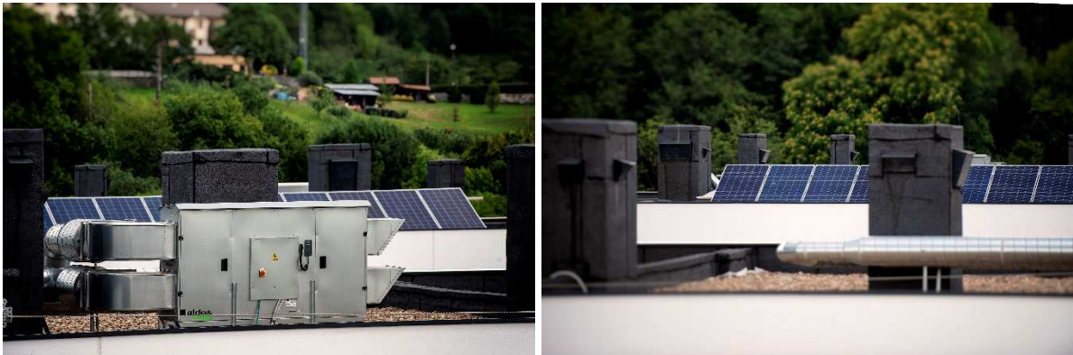
Figure 38: Heat Recovery and PV
