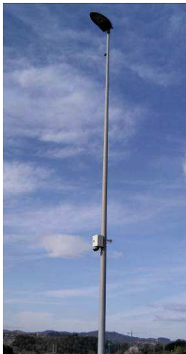
Led COB, System inside Pole, + Vision IP device, Vision detection
