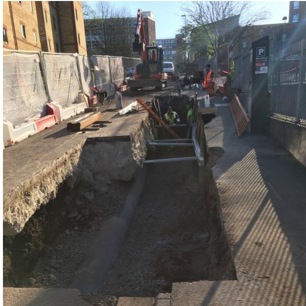
Figure 12: Trench showing existing water main
