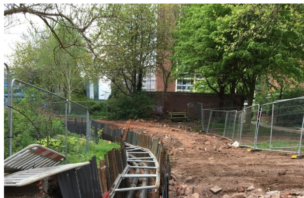
Figure 13: Trench showing pipe installation
